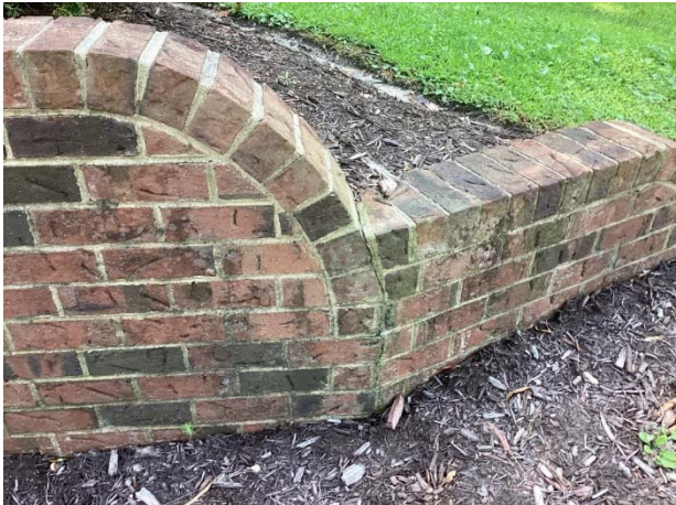
Mortar deterioration
