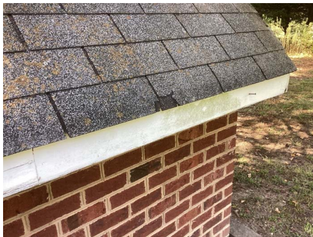
Shingle damage
